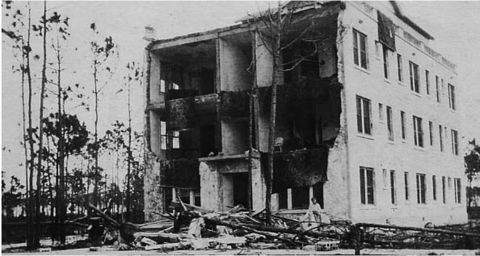
The Obispo Apartments after the 1926 storm, the front wall of 2 nd and 3 rd floor were destroyed; rugs were hung out to dry. The building was rebuilt thanks to property insurance but the Lesters lost the property during the Great Depression.
