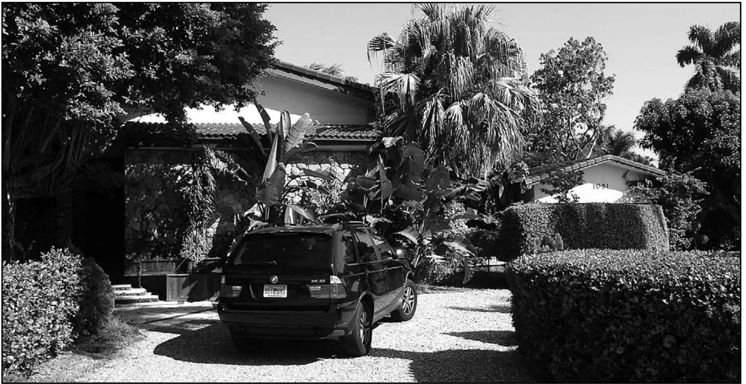
Fig. 22b – Current photo of Ritchie House showing modification inappropriate for the architectural style of the Ritchie House [photo by Louis Friend, 2006]
