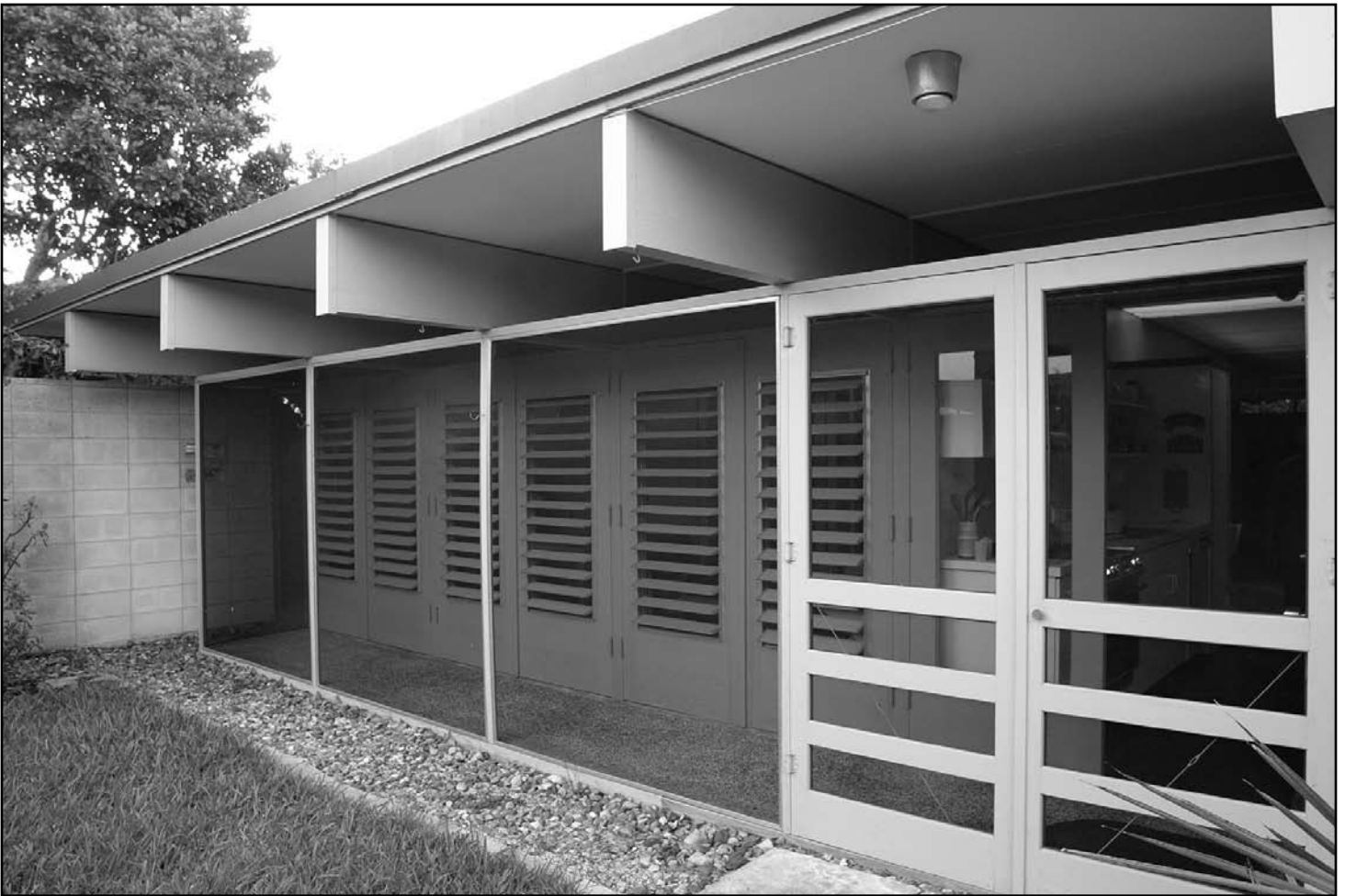
Fig. 11 – Exterior wall system of String House including louvered door and screened vestibule assemblies that address ventilation, natural lighting, and privacy [photo by Louis Friend, 2006]
