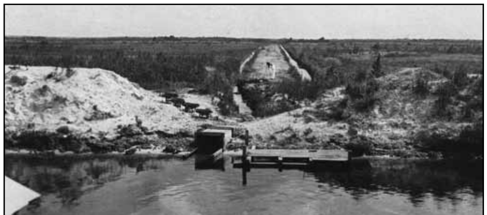
Roadbed construction, 1911. (Image courtesy the Old Davie School)
