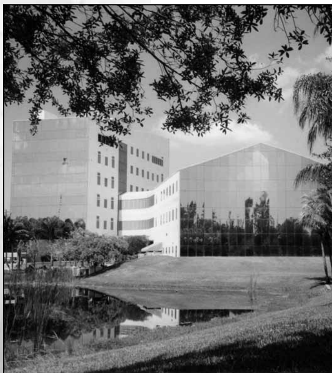
Pembroke Pines City Hall, south view 2001 (Photo by Gerry Witoshynsky)
