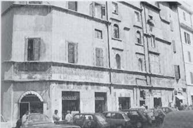
Figure 7. Casa di Lorenzo Manilio, c. 1469, Rome. Photograph courtesy of Jack Freiberg.
