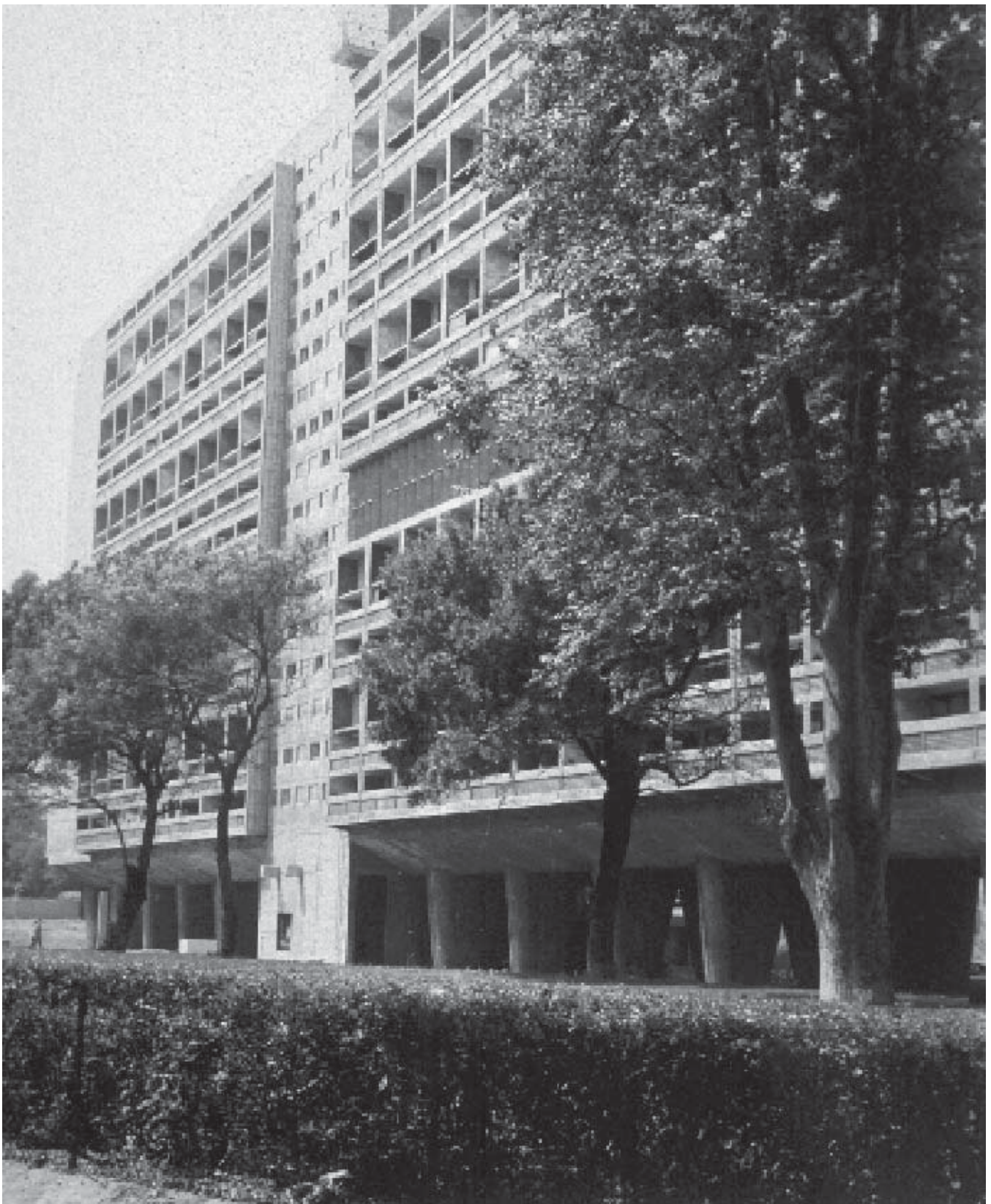
Figure 2. Le Corbusier, La Cité radieuse (Unité d'Habitation), exterior, Marseille, France, 1947-53. Credit: Giraudon/Art Resource, NY.
