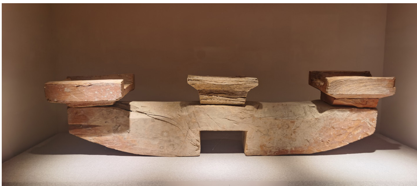
Figure 10. A bracket-set consisting of an arm and three blocks, of which the arm was discovered near Mogao Cave 130. Photo by author, May 11, 2022.
