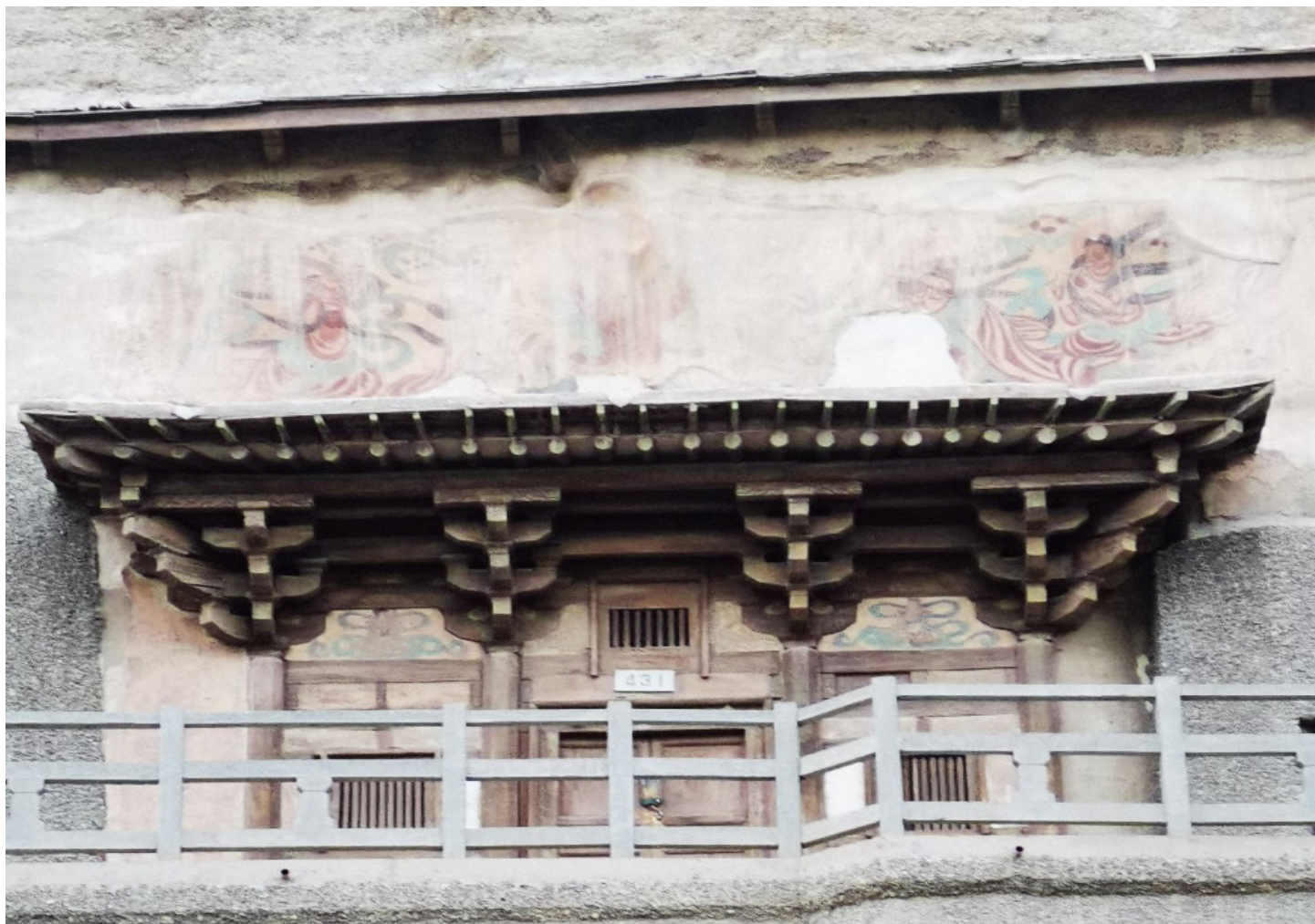
Figure 1. The timber-structured façade of Mogao Cave 431, showing three-step bracket-sets, a three-bay façade, and an overhanging roof. Dated by inscription to 980 CE. 486 cm(w) x 142 cm (d.) x 320 cm (h.). Wood, mud brick, polychromic pigments. Photo by author, January 20, 2022.
