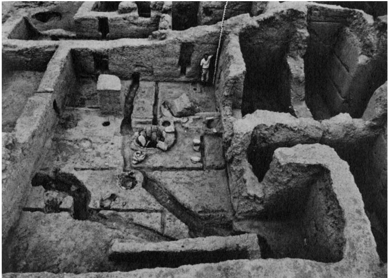
Figure 3. [below] Beneath Casas Grandes a web of channels carried water through the settlement, linking cisterns, wells, irrigation channels, and potable water. The walk-in well is notable in that it is the sole source of water in the settlement not connected to this network. Charles C. Di Peso, John B. Rinaldo, and Gloria J. Fenner, Casas Grandes: Fallen Trading Center of the Chichimeca 2: The Medio Period (Flagstaff: The Amerind Foundation, Inc. with Northland Press, 1974), p. 349. Image courtesy of the Amerind Foundation.
