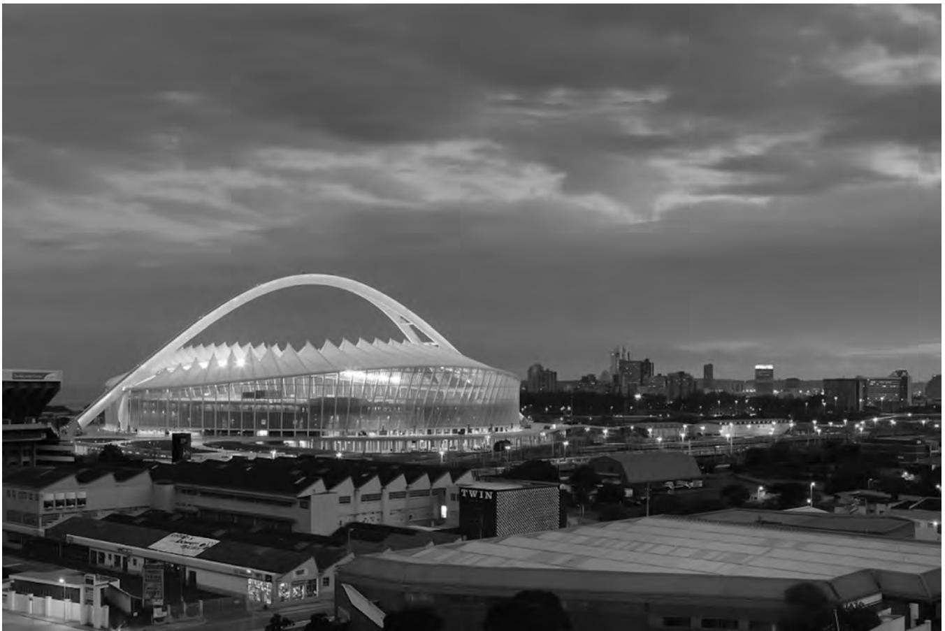
Figure 4. gmp International GmbH – architects and engineers in consortium with Ibholo Lethu Consortium, Moses Mabhida Stadium, Durban, South Africa, 2010. Photo credit: Marcus Bredt. Used by permission.
