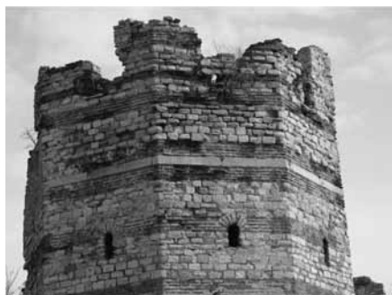
[above] Figure 1. Edirne Kapı, portal, Istanbul, Turkey c. 1453. Photo credit: Stephan Ramon Garcia.
