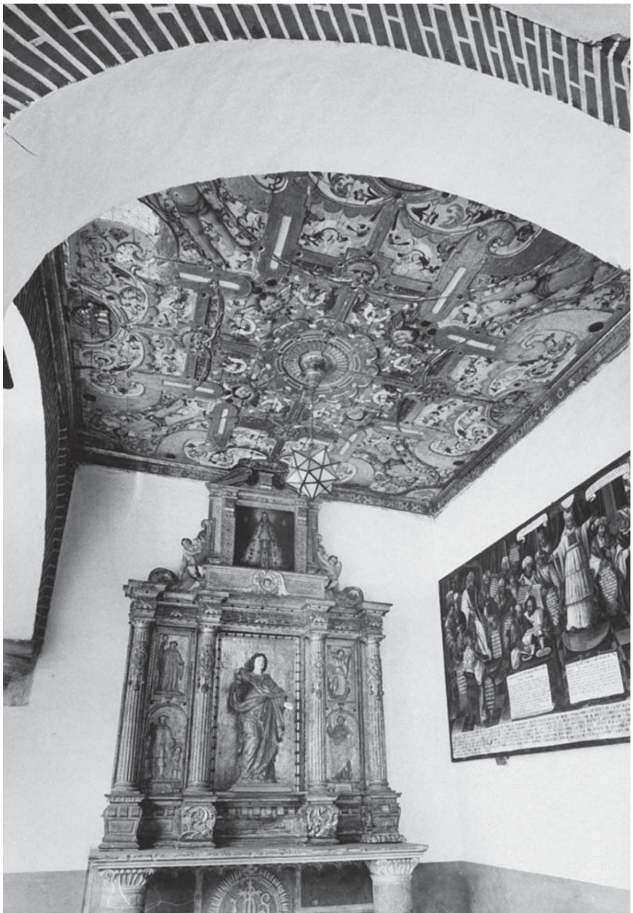
Figure 7. San Francisco, detail of lower gallery of the cloister with ceiling decoration. (Frank Scherschel - Life Magazine )
