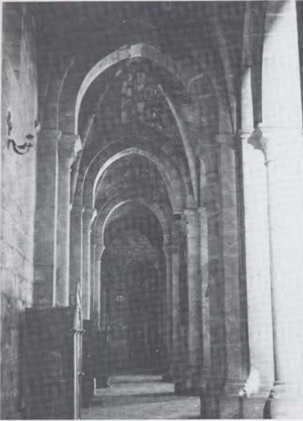
Figure 5a, Veruela. Underway 1171. North aisle of the church.
