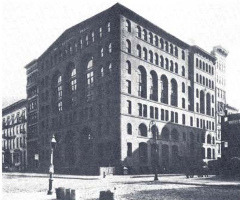
Fig. 13, Babb, Cook & Willard, DeVinne Building, New York City, 1885 ( Architectural Record , XV, 1904, 144).
