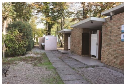
Figure 06. Photograph of Camping Fusina restrooms and the stepping up of the ground, taken by Jordan Moumne.
