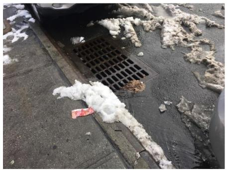
Figure 2. New York City Street Runoff from Melting Snow Entering the Drainage System. Source: Photograph by author, Flushing, New York, 2019.
